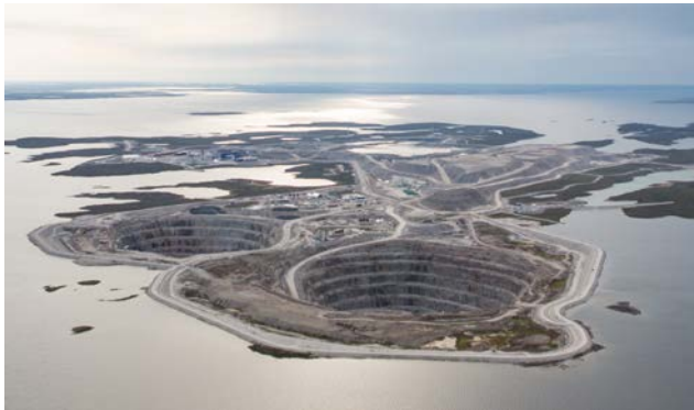
Diavik Mine, Northwest Territories Open Pit Mine (in lake) with depths in excess of 250m.
